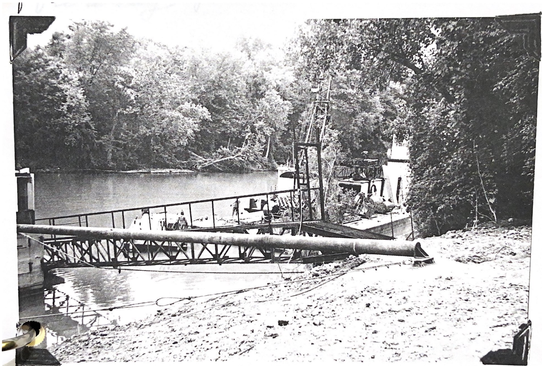
Pipes are welded into place
